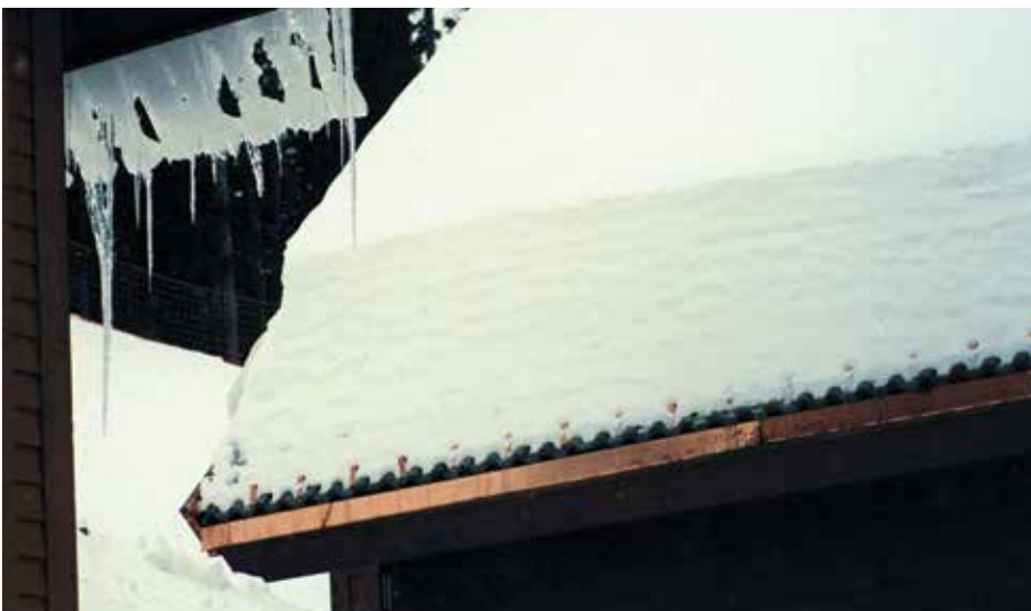
Figure 3. Cold roof system.
