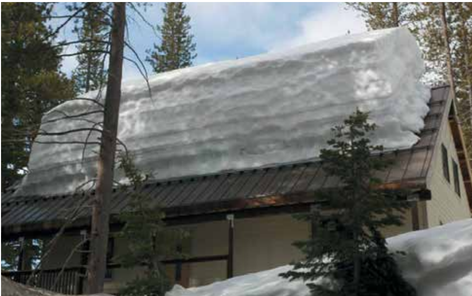
Figure 2. Snow retention on a roof.
