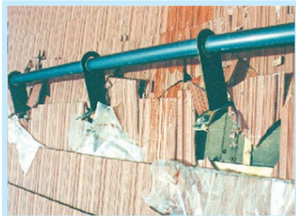
Photos 4 and 5: Snow fences used alone were not able to prevent damage.
