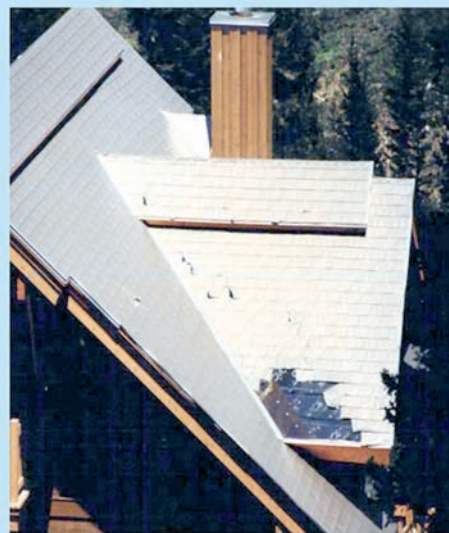
Photo 1: Damage to flat seam metal roofing.
