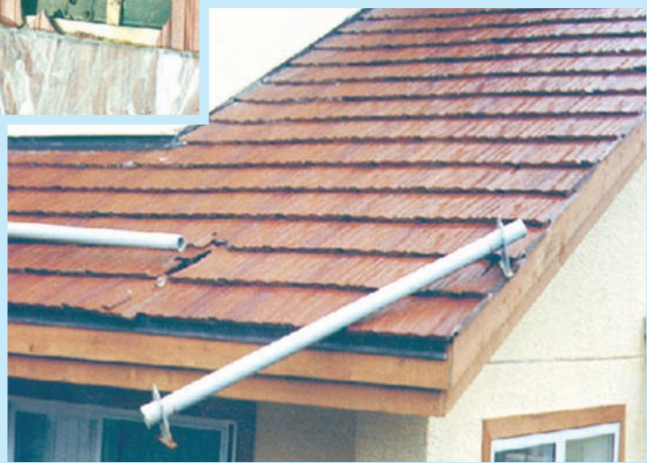
Photos 4 and 5: Snow fences used alone were not able to prevent damage.
