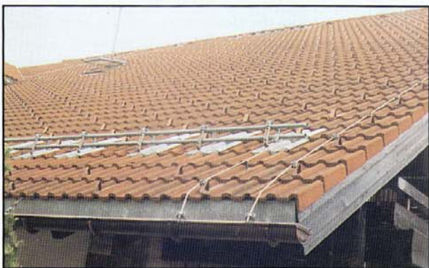
Metal snow brackets on a tile roof in the German Alps.
